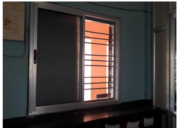
ALUMMINIUM BEADING WINDOWS REPLACED
